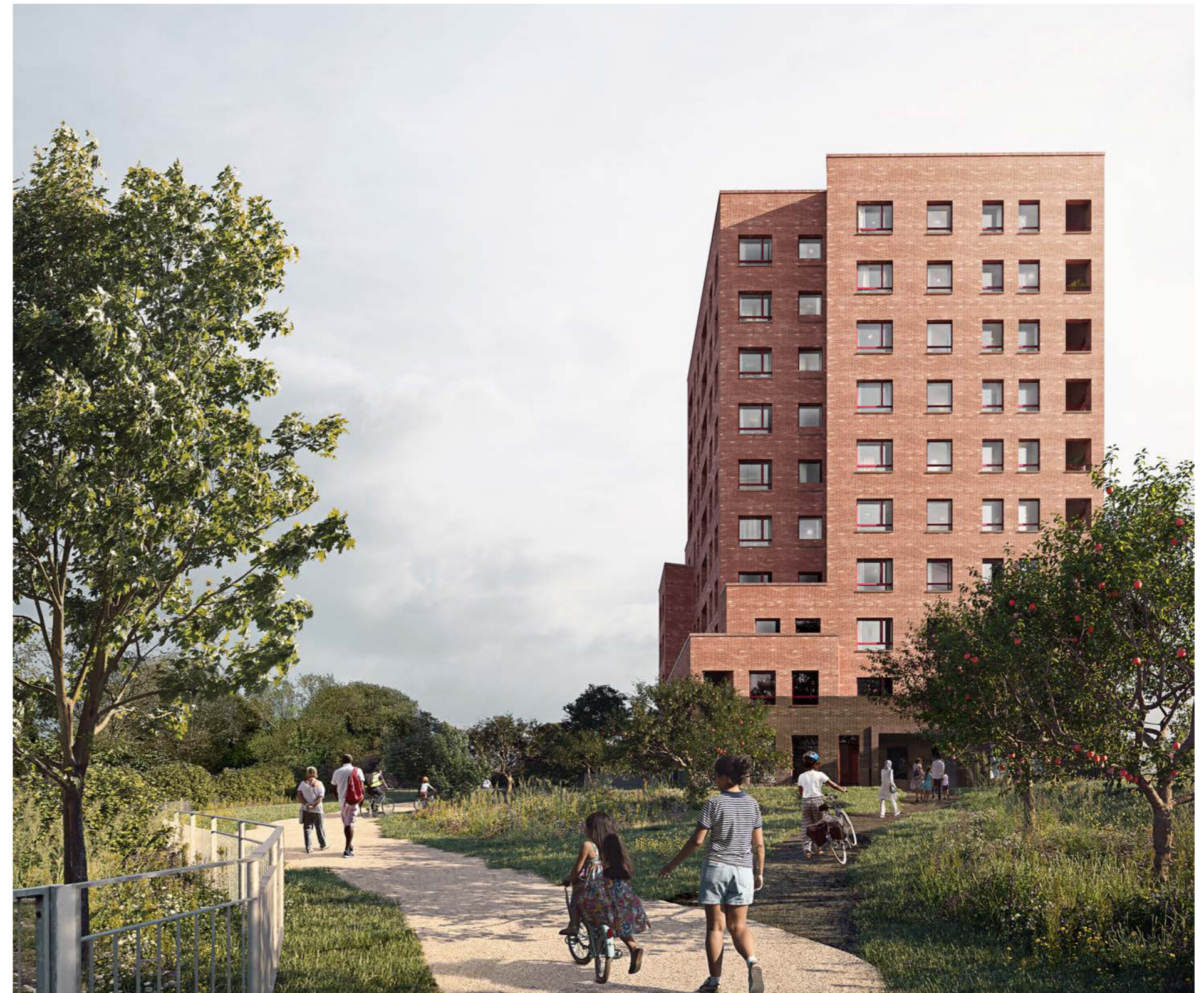
View D. View of Block A from southern park entrance from North Circular Road towards Tillett Close
