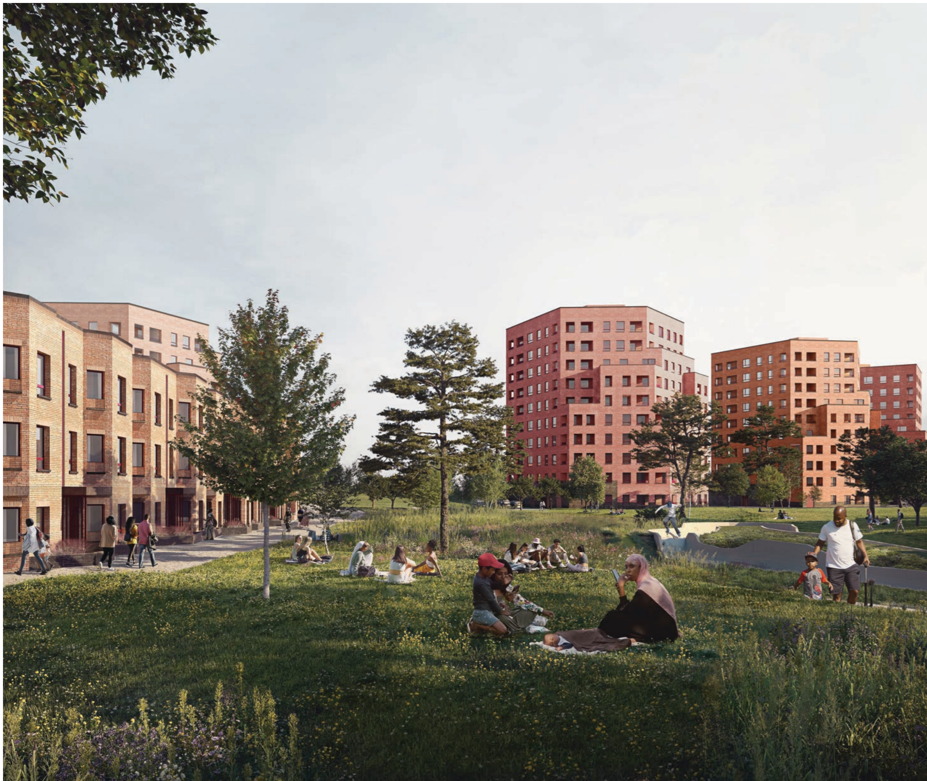
View A. Looking towards all blocks from the north of the site
